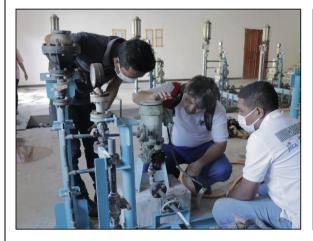
Situation of investigating a malfunctioned chemical dosing pump.
