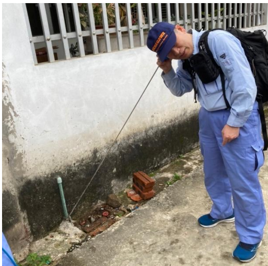
Leakage investigation in Lang
