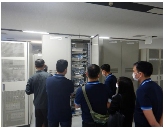
Tour of General Water Control Center
