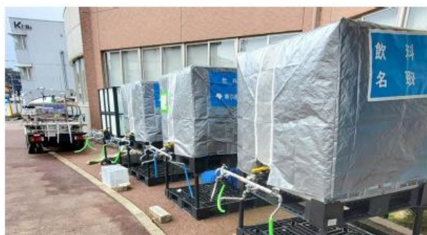
図5-25 Installation of prefabricated temporary water tanks and water supply status 38)
