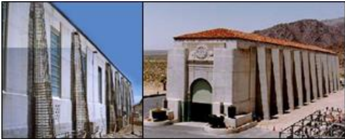
Figure 2: Seismic Upgrade of CRA Pumping Plant
