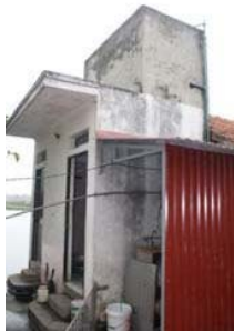
Sand filter (SF)
