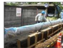
Scheduled Replacement of Water Mains (ductile pipe with anti-corrosion sleeve)
