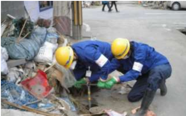
Restoring Distribution Pipes
