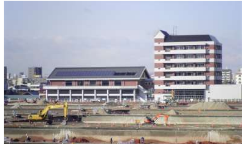
Replacement of Slow Sand Filter in Nabeyaueno Purification Plant
