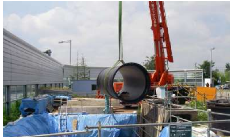
Constructing Kasugai Transmission Pipes
