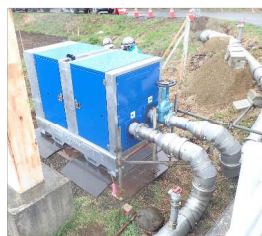
Figure 4 – The Test Run in Action
