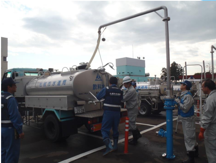
Water replenishment station(Moniwa Plant)
