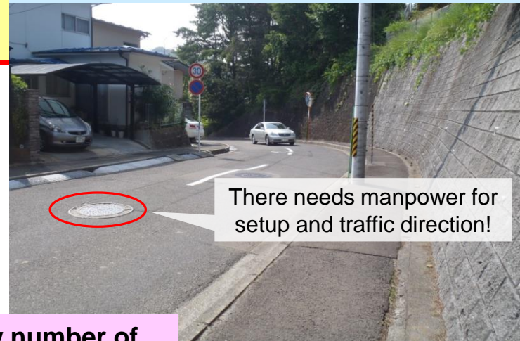
Emergency water supply facilities which were difficult to set up
